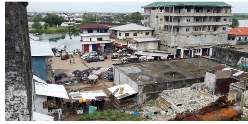
Photo 1: View on Water Street / Mesurado Estuary from Front Street
